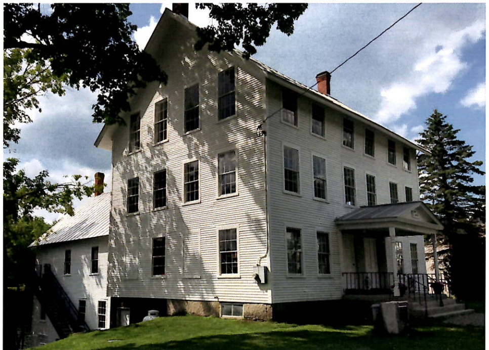
Freshly painted Old Town Hall
