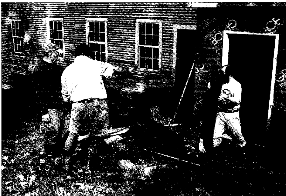
Ted Elzey, Jon Lipkovich, and Dan Childs prepare for the pouring of a concrete slab in the basement.
